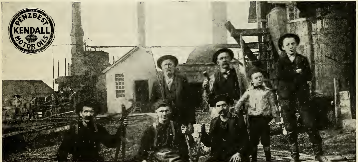
The Kendall Refinery in 1885 and its entire crew of five men—including the teamster. The white building housed the steam plant. Behind it is the “cheese box” crude still. The two-horse team and wagon was the only “pipe line” from the wells.
